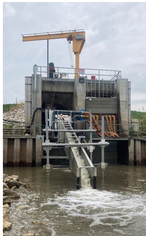
Figure 1. WHOOSH fish ladder installed at the Nature Conservancy's Emiquon water control structure near Lewistown, IL.
